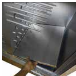
A3. Remove aluminum finishing panels
